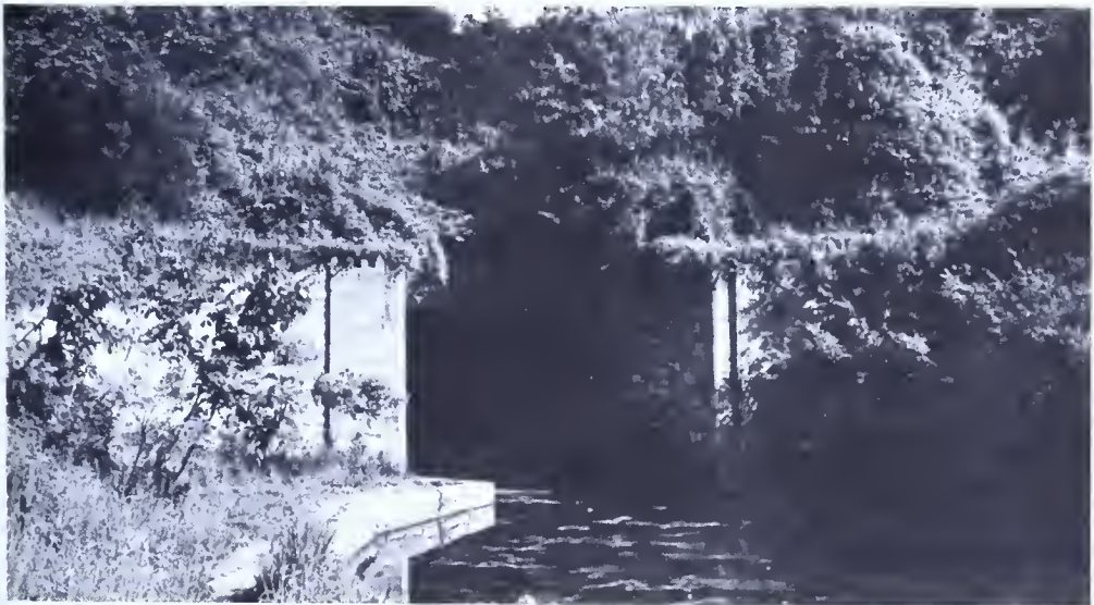
Union Canal tunnel; oldest tunnel in U.S., built 1825-1827 of local limestone and "brownstone"; North Lebanon Township, Lebanon County.
